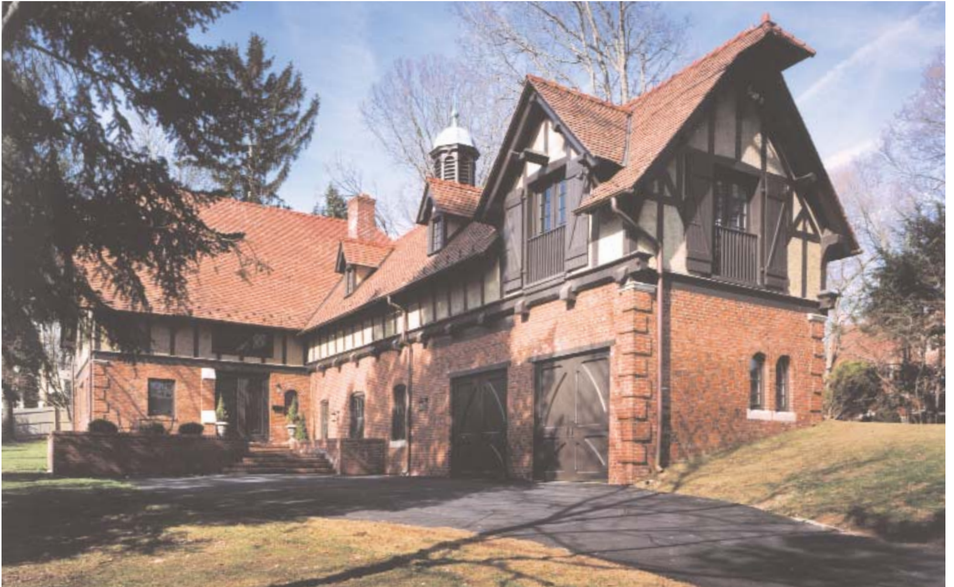
The stable at the 1898 Alan H. Reed estate, in Wayne, PA, was renovated and restored by Archer & Buchanan Architecture, Ltd., of West Chester, PA, to convert what had once been seven horse stalls, carriage bays and hay lofts into a four-bedroom home with spacious formal and informal rooms. All photos by Tom Crane Photography unless otherwise noted
