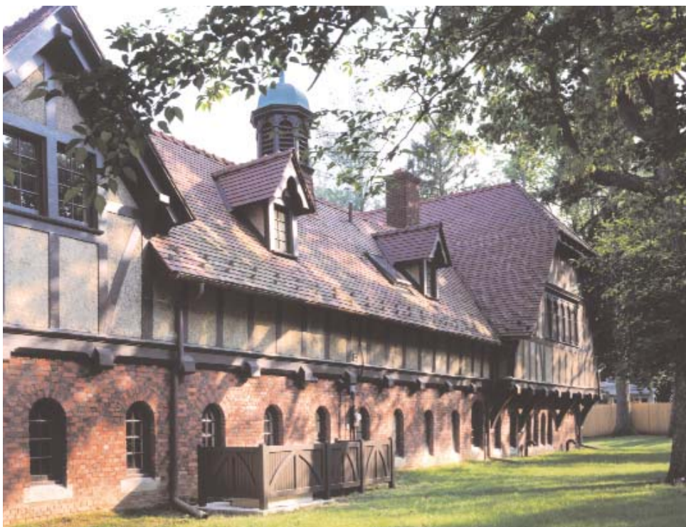
The repetitive arched window theme is reflected in other parts of the house, such as the custom muntin pattern of new French doors, manufactured by Pella Windows & Doors of Pella, IA. The removal of a second-floor window (added ca. 1960) under the main gable restored the original symmetry of the façade.
