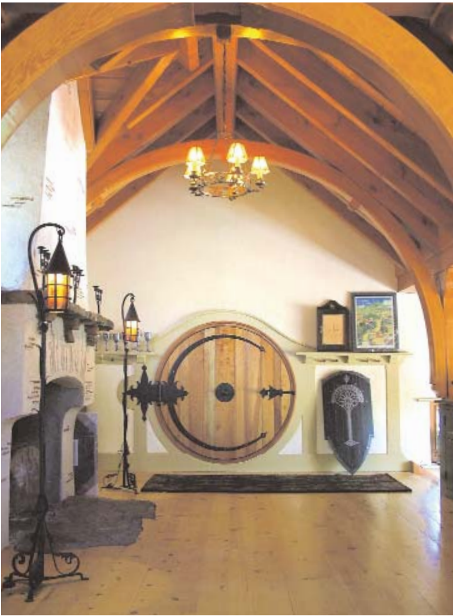
The interior of the Hobbit house, replete with Tolkien memorabilia, is accessed by a 54-in.-dia Spanish cedar door adorned with a hand-forged, single-pivot hinge.
