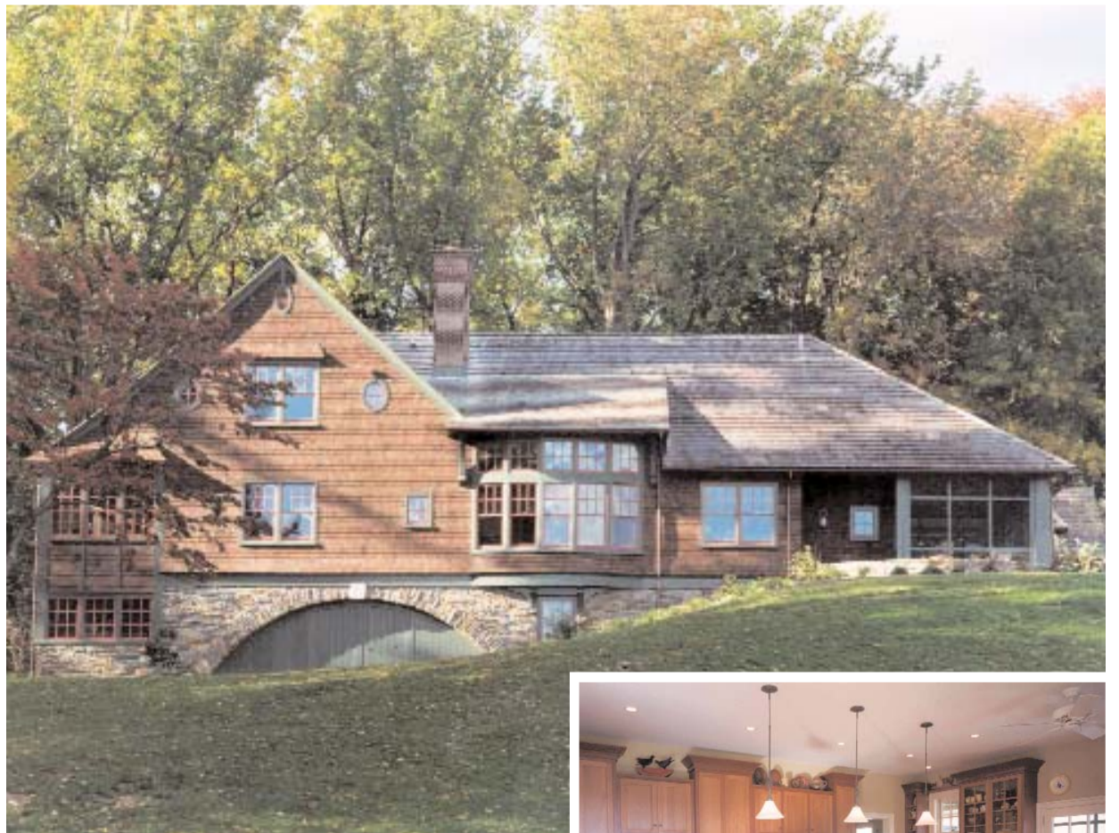
Above: In West Chester, the firm designed a 5,100-sq.-ft. Shingle-style residence in 2001. Characterized by a number of shed dormers and heavy bracketing, the design conforms to its setting – the slope of the site allowed for a 26-ft.-wide stone archway leading to a basement garage.
