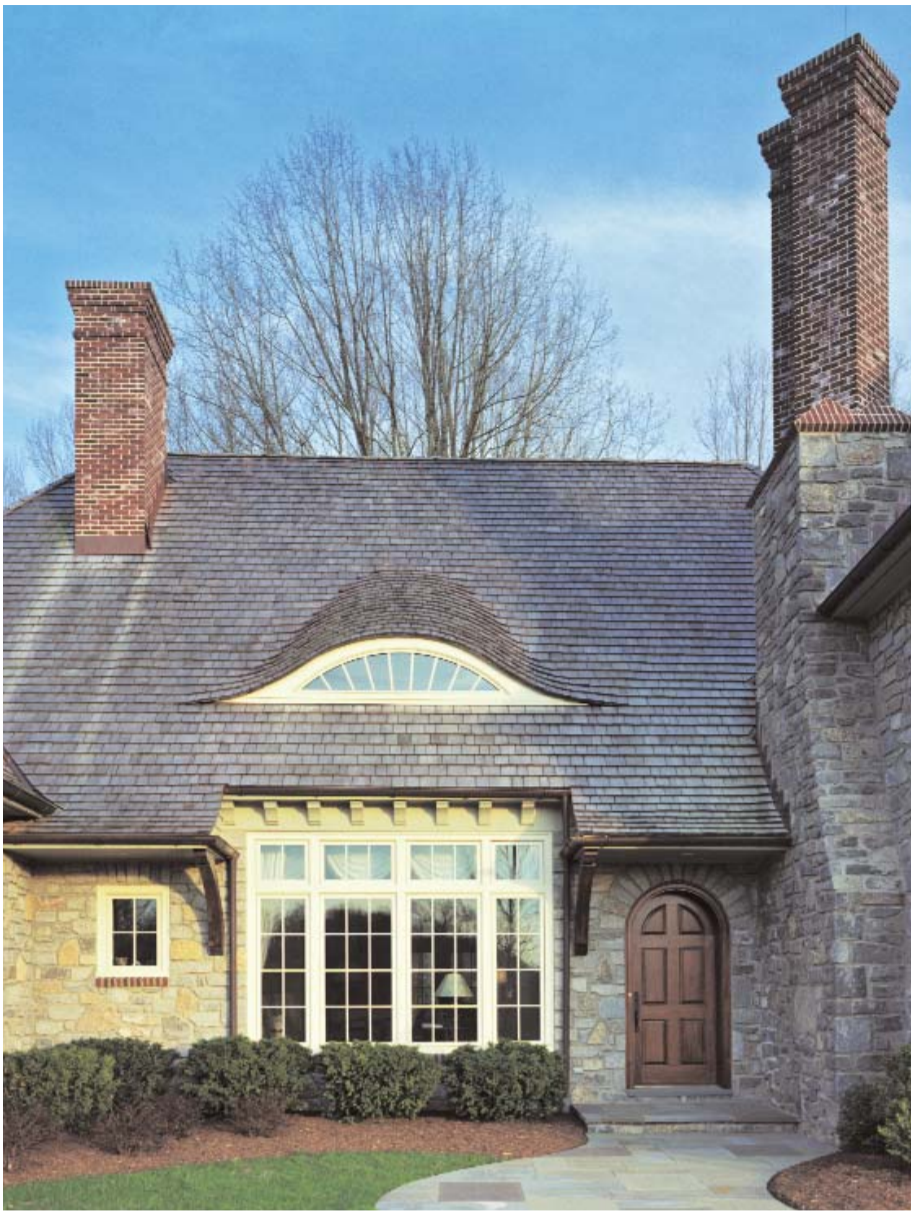
A stone house in Greenville, DE, was based on English and local precedents. The extensive fenestration requested by the client is offset by the stonework and heavy roof.
